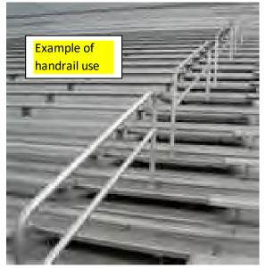
• **Handrails**—Consideration should be given to the installation of handrails in the aisles.
