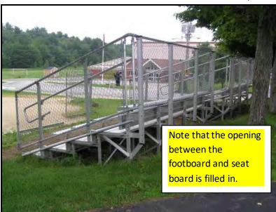
• There should be no more than a 4inch gap between the guardrail and the seat or footboard. In addition, there should be no more than a 4 inch opening between components of the guardrail.
